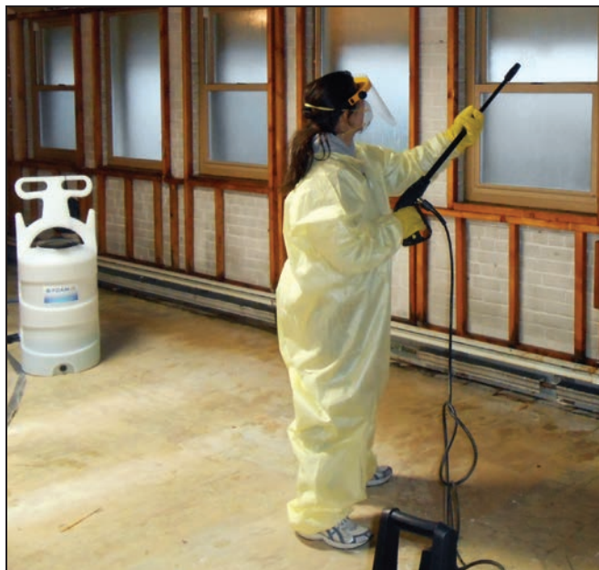
Figure 3. Using a pressure washer to rinse surfaces cleaned with a foam solution
